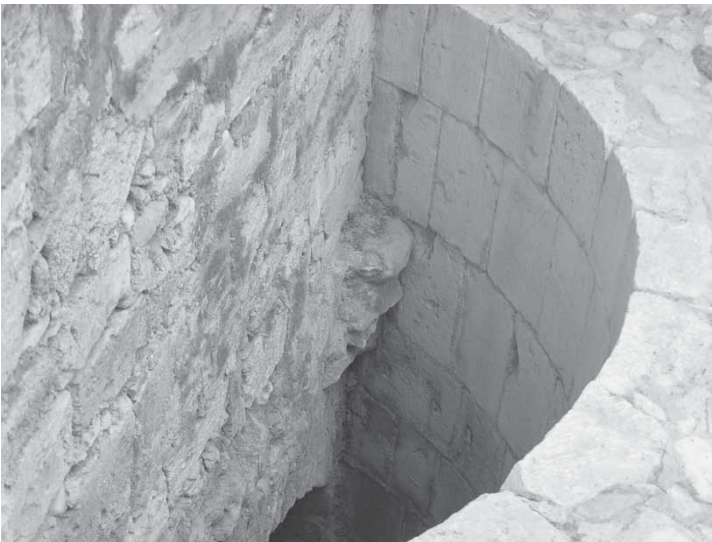
Fig. 57: Limassol, Great Mosque, south apse, detail of fragment of plaster floor attached to the eastern wall of the present building [M. Olympios].
